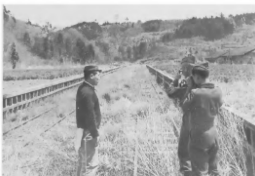
Figure 20. These rail lines once brought the envelopes, manitons, and other supplies needed to operate the balloon offensive at Otsu. (U.S. Army photograph, SC 283910-5)
